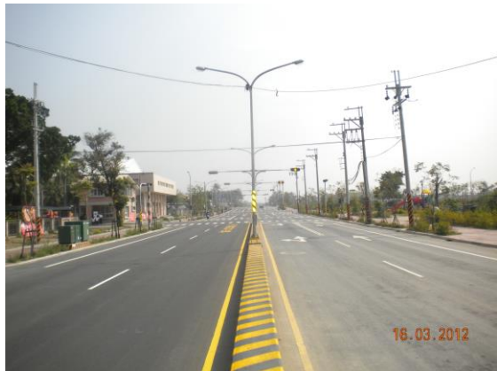
(c) 0K+400~0K+958 路面竣工
