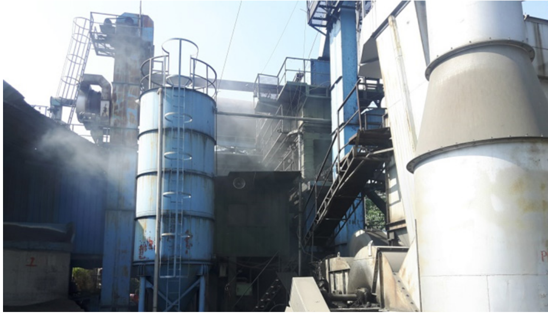
▲ Mixing asphaltic concrete is a major air-polluting act.
