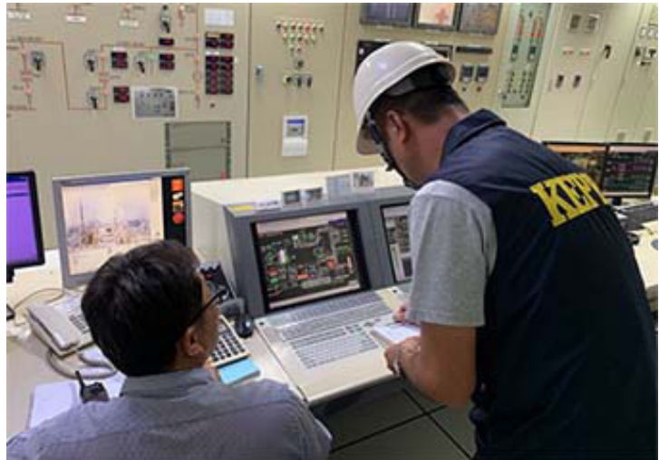
▲ Onsite plant inspection
